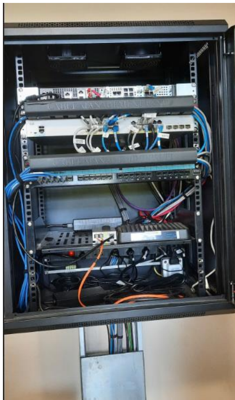
Figura 3.1 Tablero VSAT (Rack)
